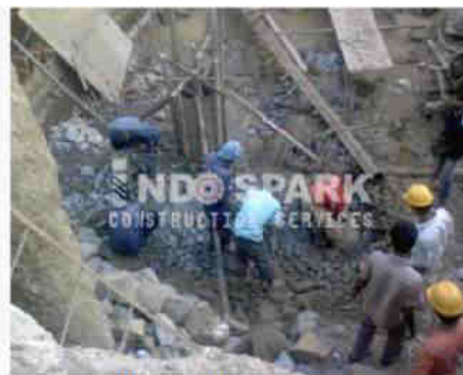
Pile Breaking at Mumbai
