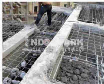
Breaking of Water Tank at Undri, Pune
